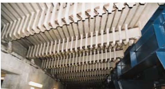
Fig. 48: Few from underneath in the abutment on the control mechanism of a installed DS 2000 (Storebaelt Bridge, Denmark)
