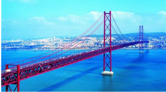
Fig. 42: Tejo Bridge in Lisbon fitted with a DS seismic expansion joint
