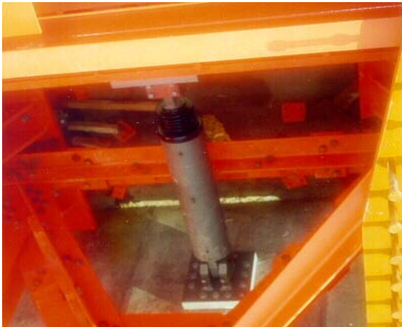
Fig. 37: Sample for anchoring of MHD to abutment
