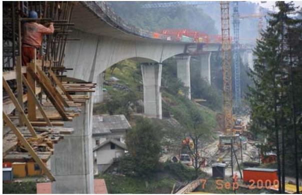
Fig. 33: Twin Viaduct Locica in Slovenia with MHDs
